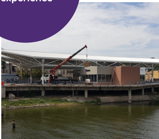
Construction at Elgin Transportation Center
