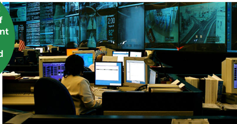
CTA Control Center
