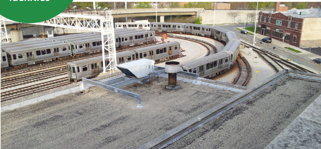
Rail Shop roof and mechanical equipment
