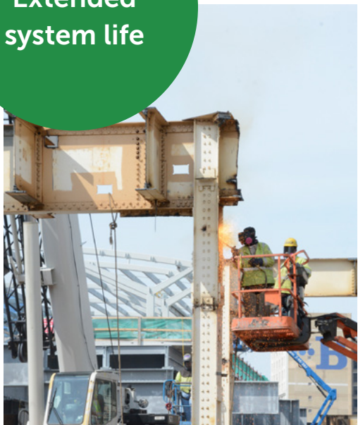
Elevated steel structure renewal
