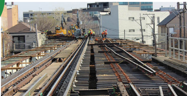
Brown Line elevated trackwork
