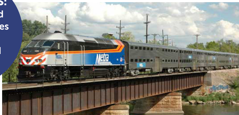
Milwaukee District-West Line bridge over Fox River (replacement currently underway)
