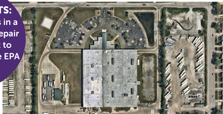
Pace South Division Garage with new CNG fueling station (Located in Markham, IL)
