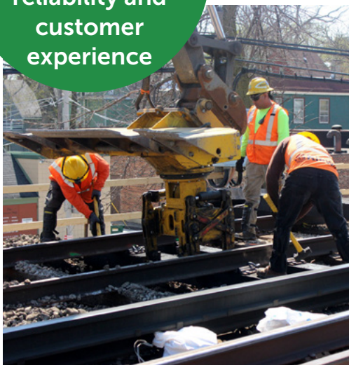
Green Line trackwork
