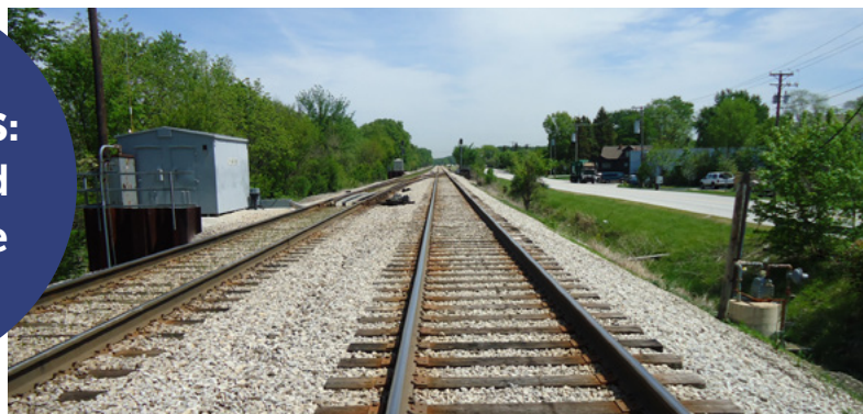
Mainline track on Rock Island for 79 mph operation
