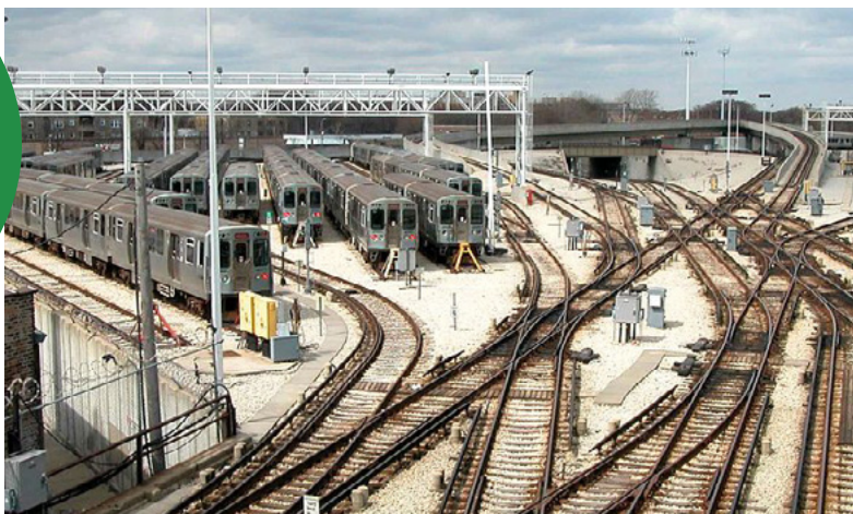
Complicated track work at Howard rail yard
