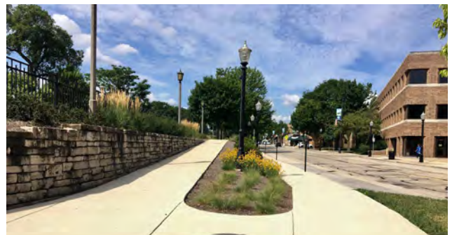
ADA-accessible ramp, pedestrian lighting, and landscaping at train station
