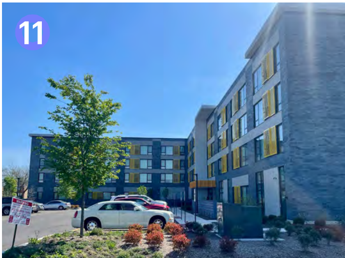
Placing parking behind buildings activates and frees up the frontage for pedestrian-oriented features
