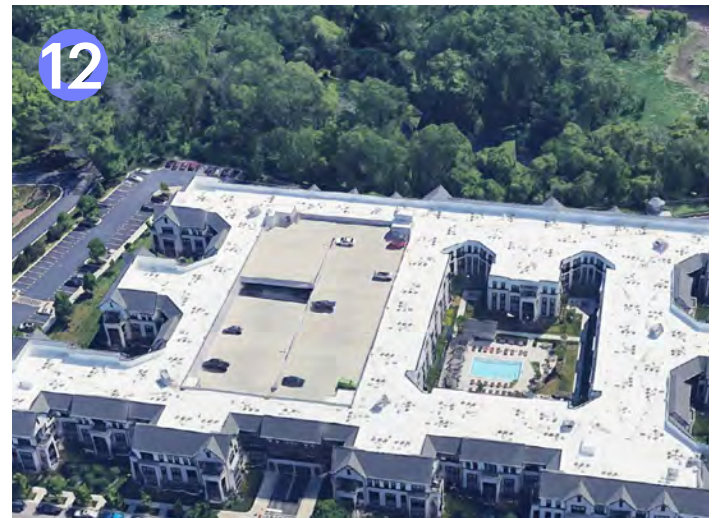
Wrapped parking refers to a parking structure that is wrapped/hidden by other uses facing the street frontage.
