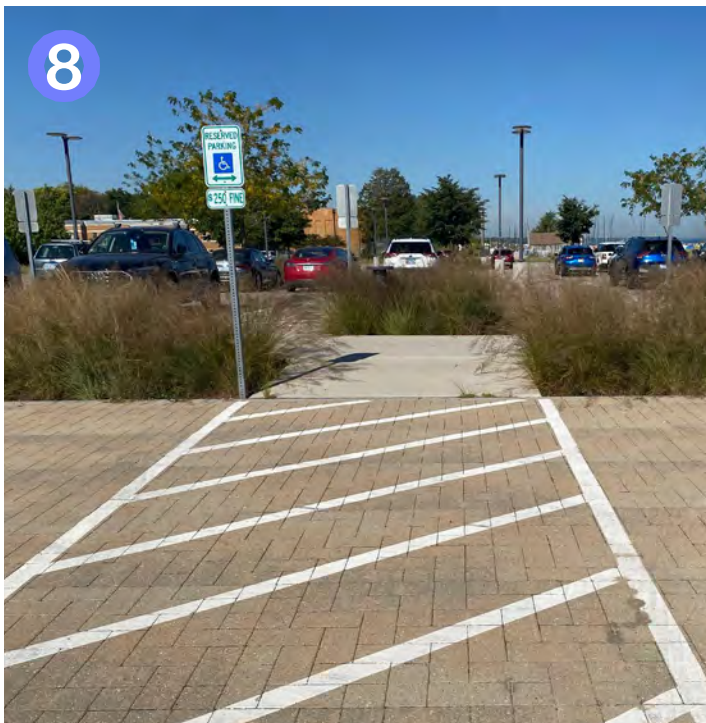
ADA accessibility is enhanced with sustainable design, such as pervious pavers and native plantings.
