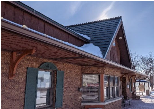
Existing Fox Lake crew facility.
