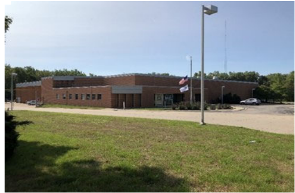
Existing River Division Garage.
