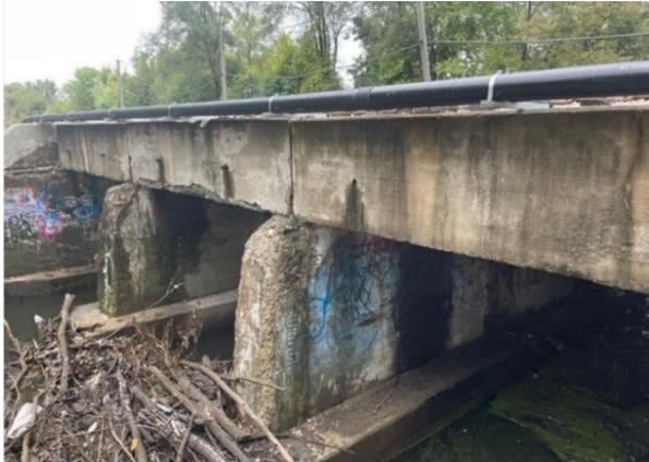
Current condition of the Stoney Creek Bridge.
