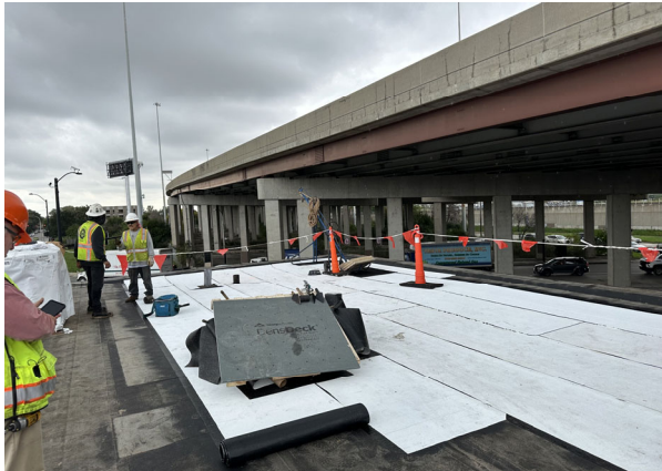
Contractors working on the substation roof replacement.
