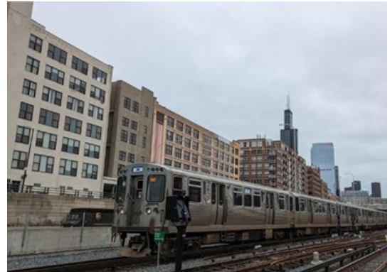
Photo taken during the final walkthrough of the track replacement on the Forest Park Branch.
