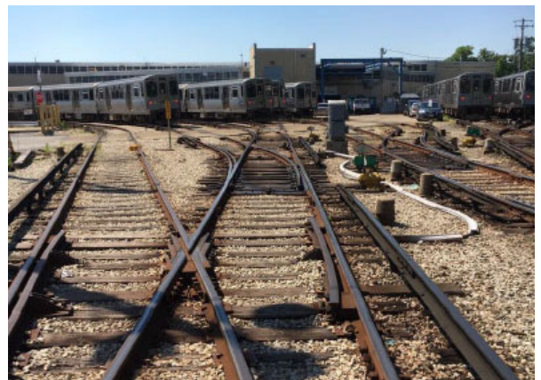
Existing Track at Des Plaines Yard.
