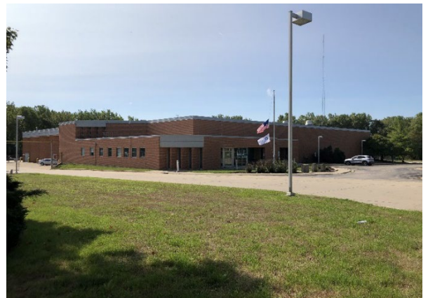
Existing River Division bus garage.
