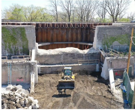
Construction activities at the new Metra Auburn Park Station.
