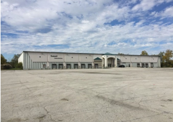
Current photo of the warehouse building.
