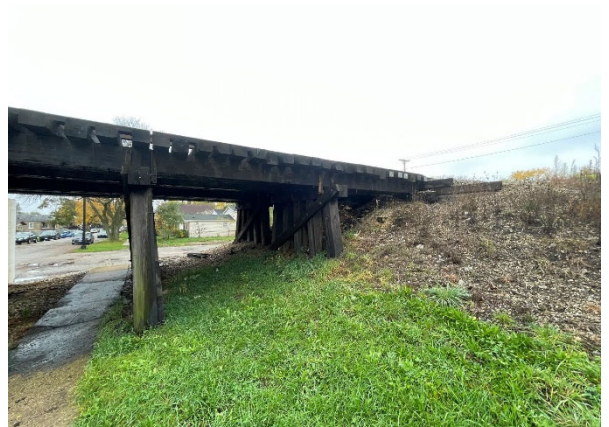
Current photo of Morgan Street Bridge.
