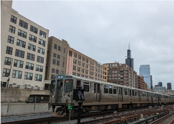
CTA Blue Line train on the new track close to Racine Street.
