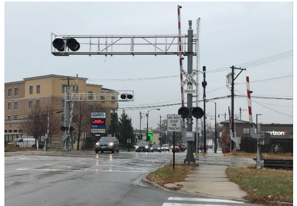
Existing Metra grade crossing.
