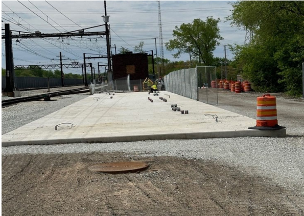
Construction activities at the Matteson Substation project site.
