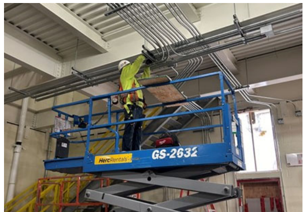
Damen Substation Interior Electrical Installation.
