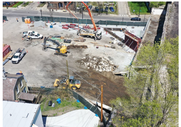
Construction activities at the Auburn Park Station project site.
