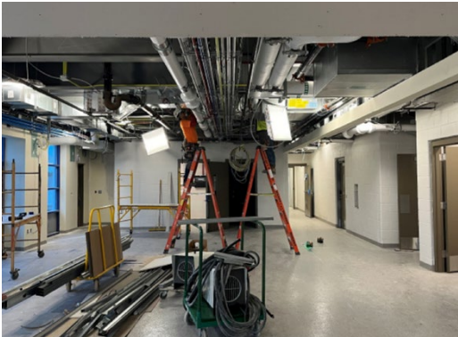
Acceptance Facility framing installation.
