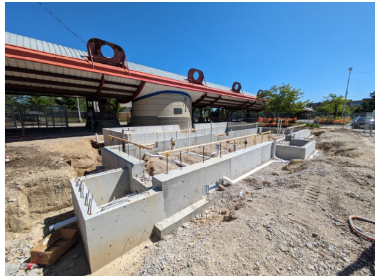
Poured foundation and underground utilities for the new ADA Transfer Center.
