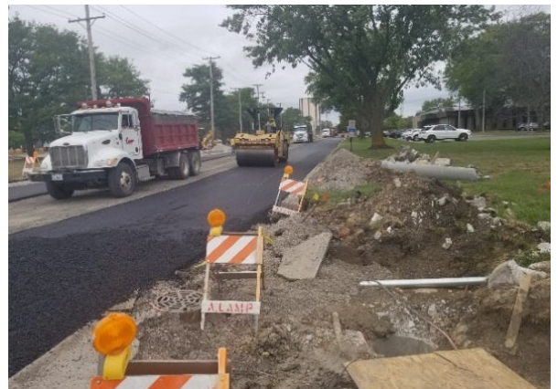
Improvements to Old Willow Road.
