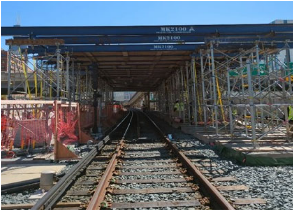
Scaffold framing and bracing at Racine.
