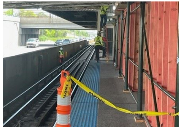
Canopy demolition at the Harlem Station Bus Bridge project.
